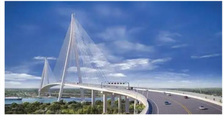
North America's longest cable-stayed bridge at a price tag of $6.4 Billion.
